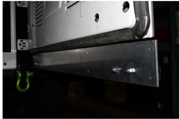
Using the provided 5/16" nuts and bolts, attach the bottom of the hinges to the bottom aluminum panel. Once the bottom panel is installed the backside of the nuts will not be accessible.....so tighten them securely and use grease to prevent the bolts from galling.
